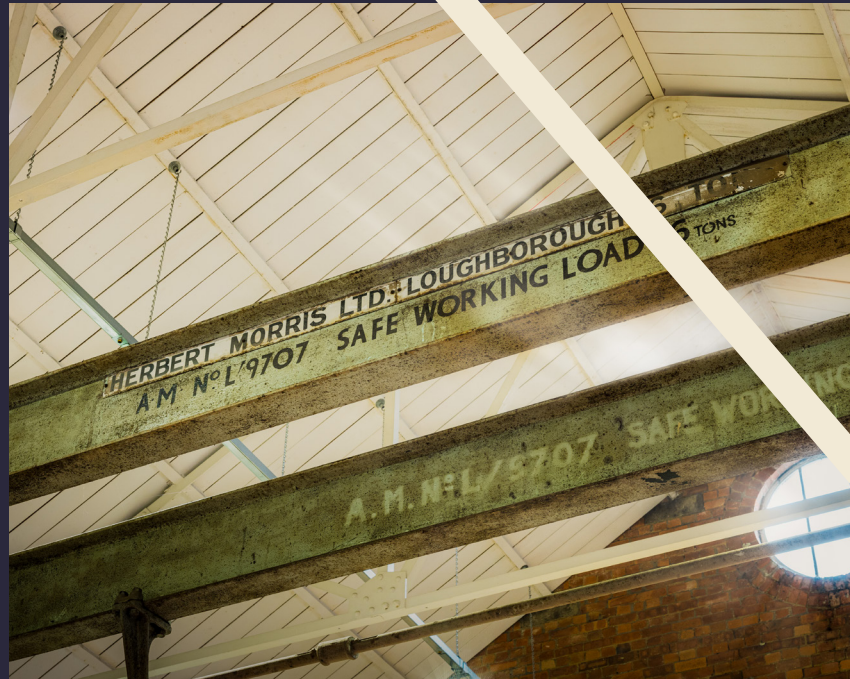
The Power House retains its original Air Ministry beam crane.
